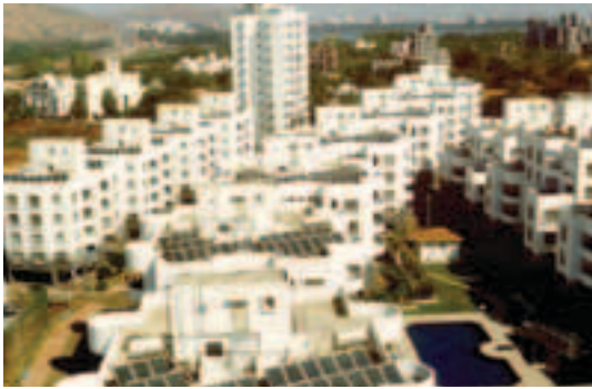
Figure 8.4 Solar water heater system 2
